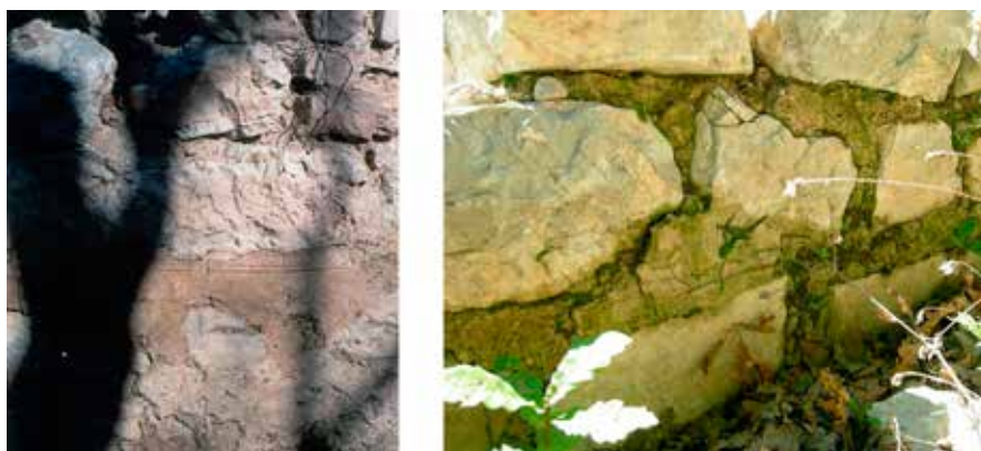
Fig. 5. Remnants of mortar-filled joints and horizontal lines drawn in fresh mortar on the outer face of the central apse (photo: J. Šurdilović, 2002; archives of the Institute for the Protection of Cultural Monuments, Niš) and of the north wall (photo: author, 2006)
